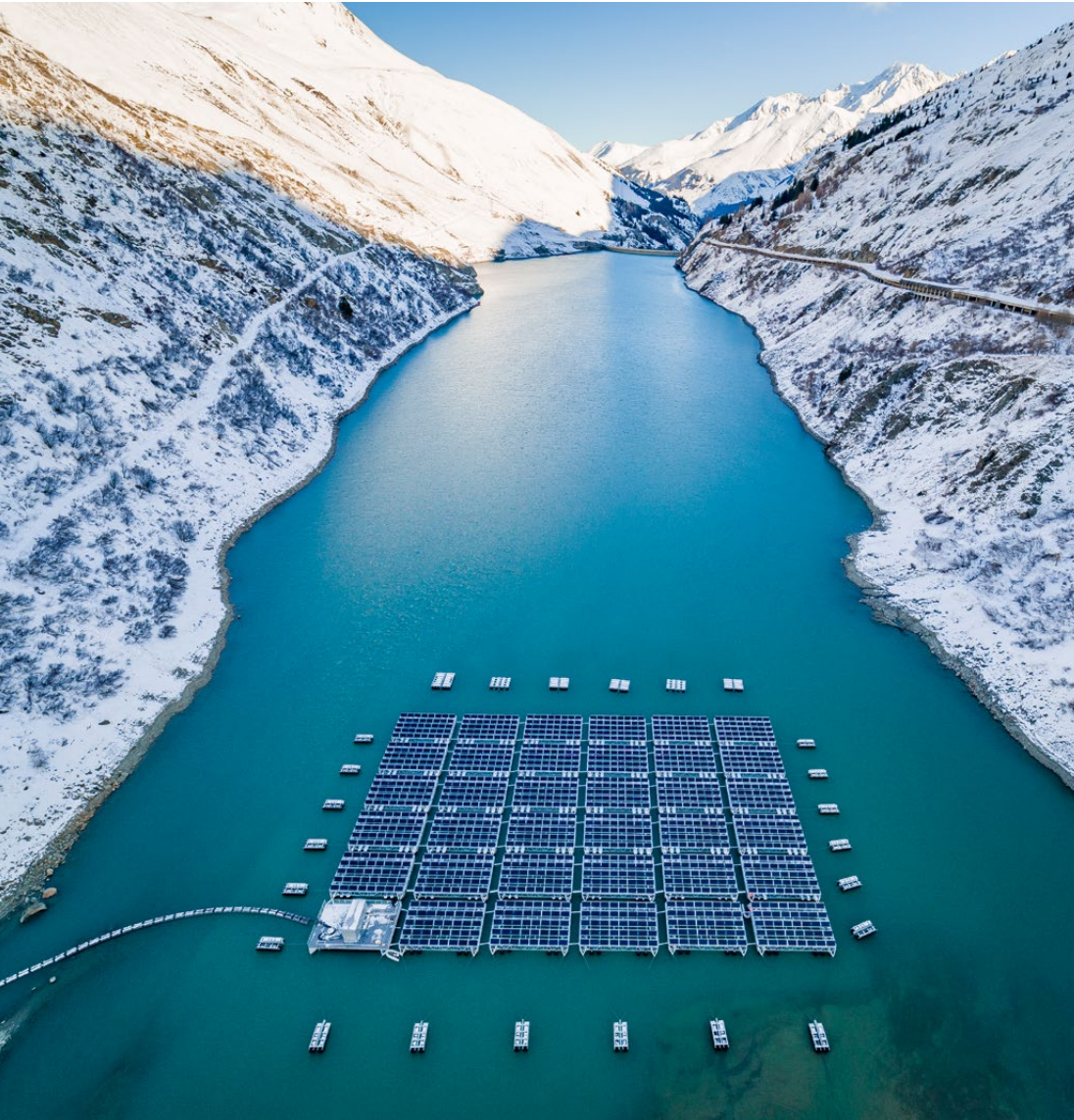
Source: Romand Energie. Floating solar farm on Lac des Toules, in the Valais municipality of Bourg-Saint-Pierre.
